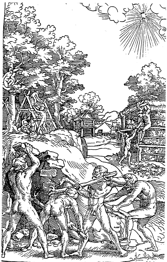
Fig. 1 Illustrations proposed for Marcus Vitruvius Pollio's Architectura Libri Decem , edited by Ryff, 1548.
